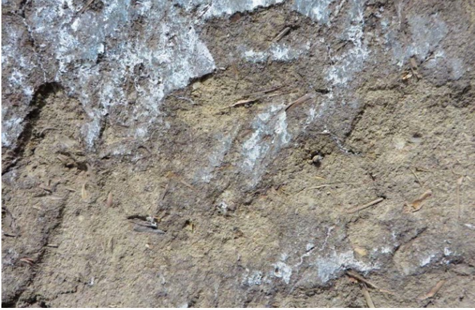
One of the adobe bricks inside the cocina. One can see the straw that was included in the adobe mixture.
